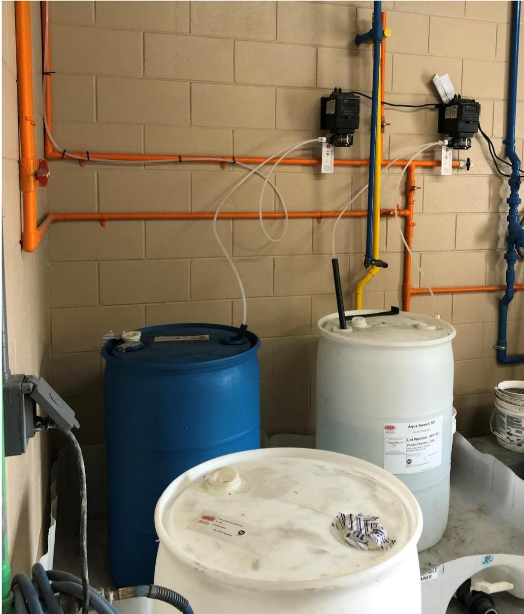
If the polymer system is to be continued, a replacement system is recommended. Installing a neat polymer mixing and dosing system would allow the city to use neat polymer and eliminate the need to mix and/or dilute dry or bulk liquid polymer.
