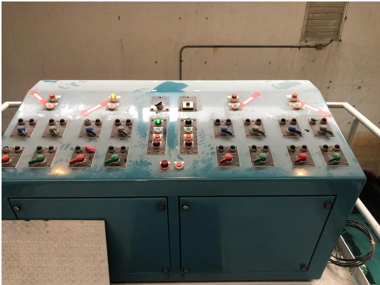
Overall, a complete rehabilitation of the control system is warranted to provide necessary operator control, remote management, and to reduce the burden on operational staff.
