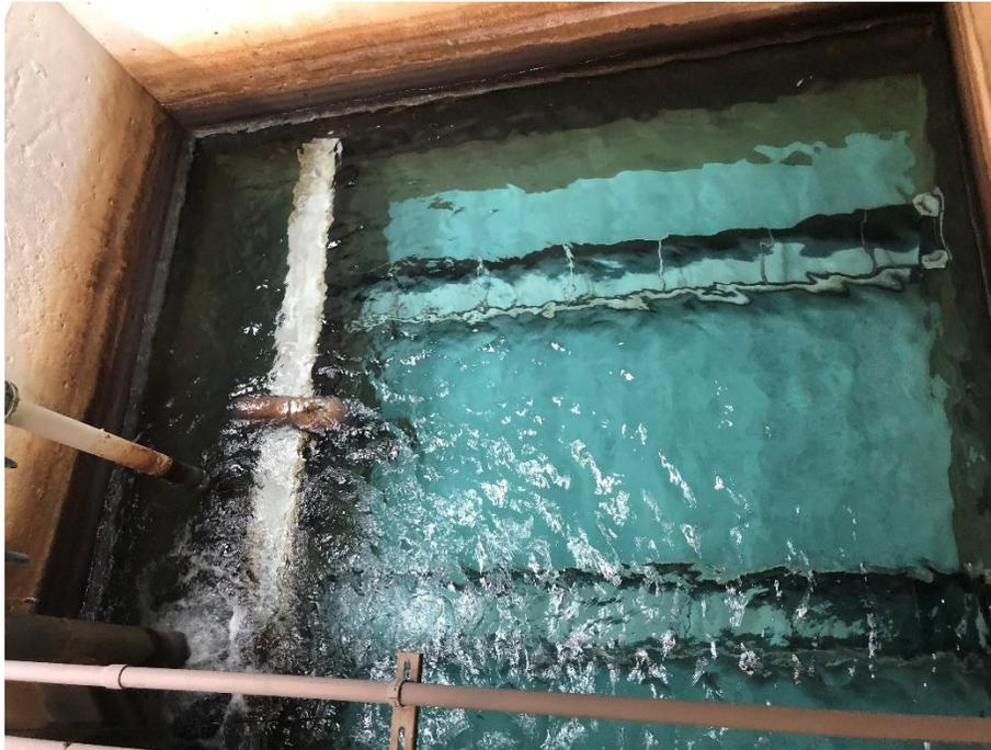
The filters consist of 18" of anthracite media (0.6 to 0.8 mm), 12" of sand (0.5 to 0.6 mm), and support gravel. According to available information, the filter media was last replaced in 2006 with filter sand (0.45 to 0.55 mm) and anthracite (0.9 to 1.0 mm). The underdrains are reported to have been replaced in 2006. The original fiberglass wash troughs are still in use.
