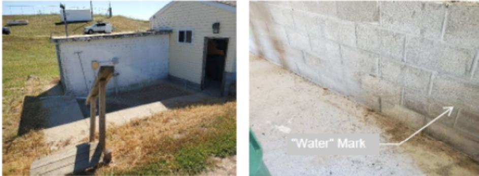
**Figure 2: Headworks and Pump Building Exterior, Wet Well (left) and Headworks High Water Mark (Interior; right)**
